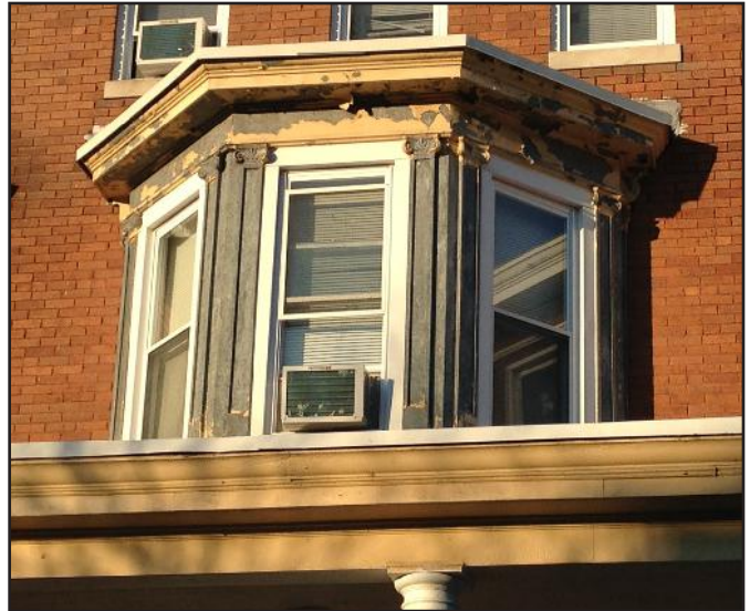
Figure 16: NOT RECOMMENDED - A metal bay window with peeling paint, but in otherwise good condition. If this remains unpainted the metal will deteriorate.
