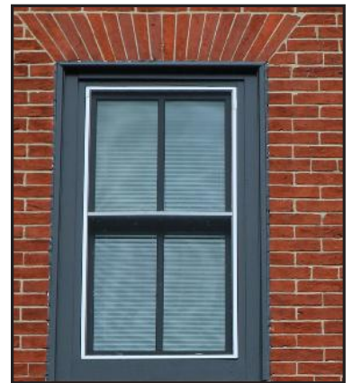
Figure 27: NOT RECOMMENDED An example of a replacement window that is too small for the historic masonry opening.
