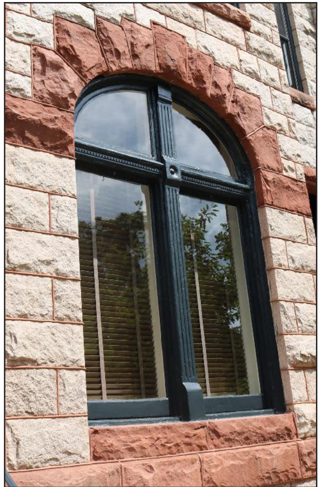
Figure 24: RECOMMENDED - Example of appropriate repair of historic wood window.
