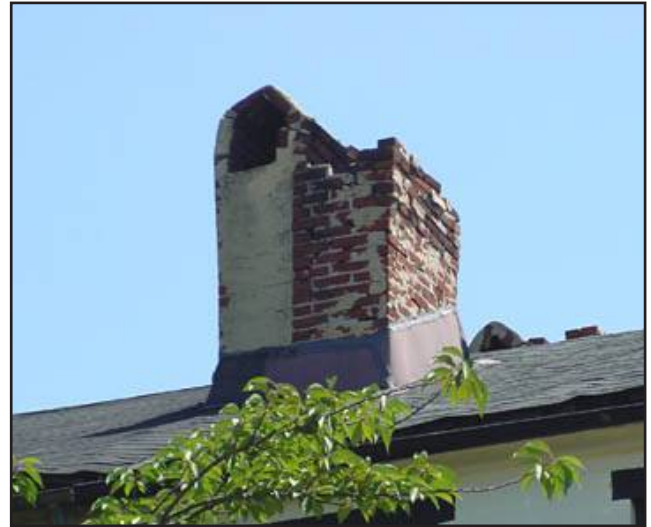
Figure 30: Example of chimney deterioration.
