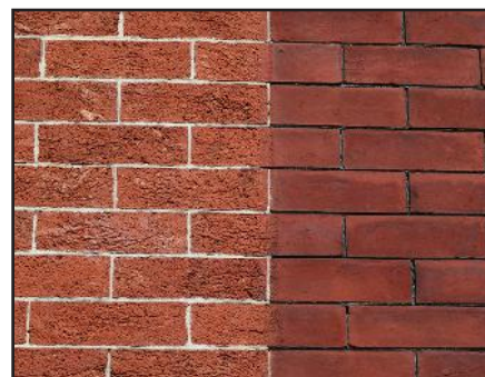
Figure 2: Adjacent properties showing the difference between brick that has been sandblasted (left) and intact historic brick (right)
