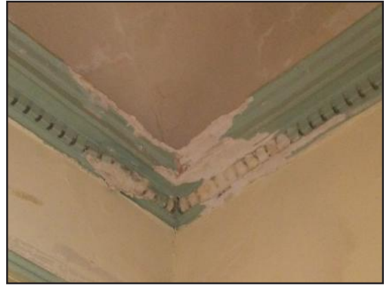
Figure 61: Deteriorating decorative plaster trim.
