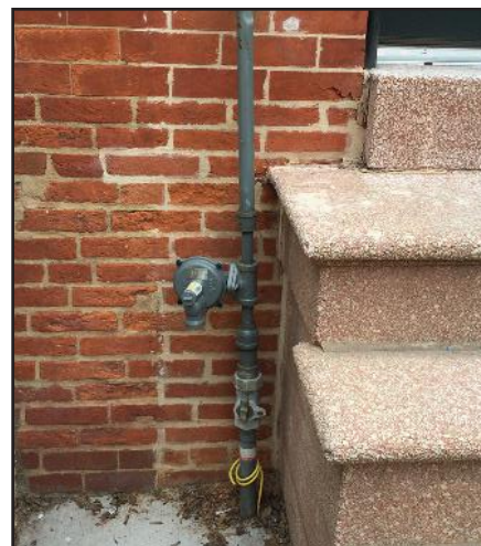
Figure 1: NOT RECOMMENDED - Example of brick wall with deteriorating mortar, water damage, and inappropriate repointing.
