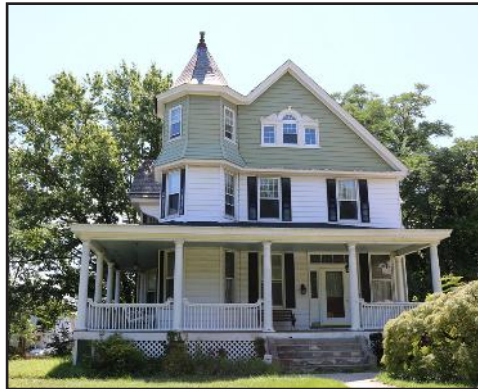
Figure 13: NOT RECOMMENDED - Use of vinyl siding over historic wood siding.
