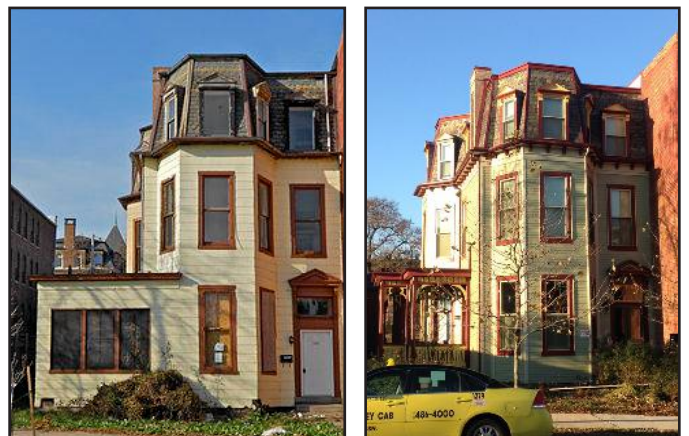
Figure 19: RECOMMENDED - The renovation at the Gertrude Stein House utilized fiber cement siding and PVC trim details to recreate the historic wood siding and trim, which was missing at the time of the renovation.
