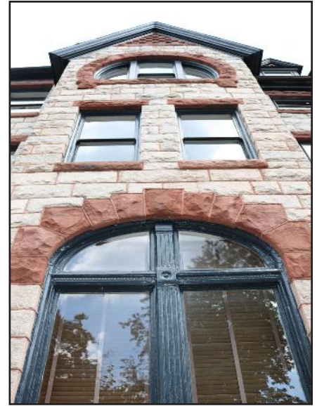
Figure 9: RECOMMENDED - Repointing of stone using appropriate mortar.
