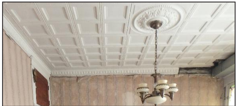
Figure 55: Example of damaged historic tin ceiling and light fixture.
