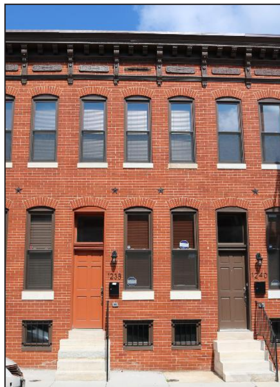
Figure 5: RECOMMENDED - Repointed brick that replicates the color, texture, composition, and tooling of the historic mortar.
