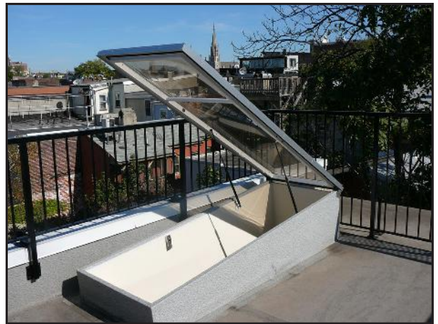
Figure 31: RECOMMENDED - Low-profile roof hatch that is not visible from street.
