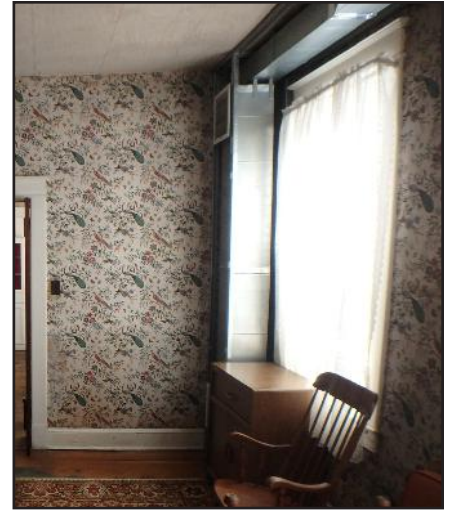
Figure 59: NOT RECOMMENDED - Inappropriate duct work in historic house.
