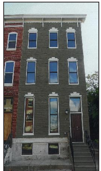
Figure 39: RECOMMENDED - Painted formstone is permissible, though not required.
